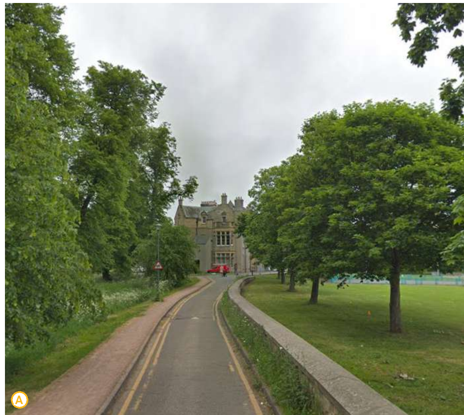
Views towards the west facade of Inch House from the historic access route. The view is framed by mature lime trees on the left
