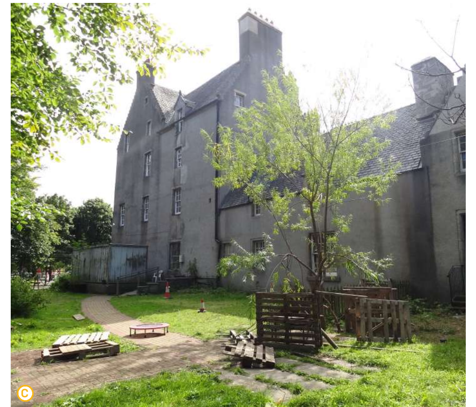
Close view of Inch House from the east. Ancillary storage detracts from the view
