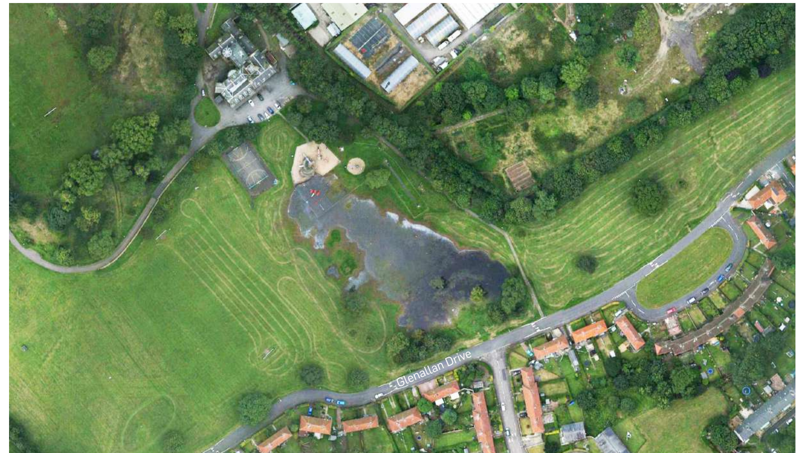
Extensive surface water flooding to the south of Inch House
