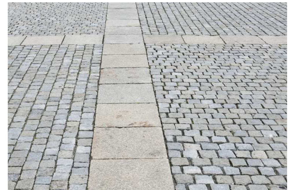
Caithness paving to cafe courtyard areas
