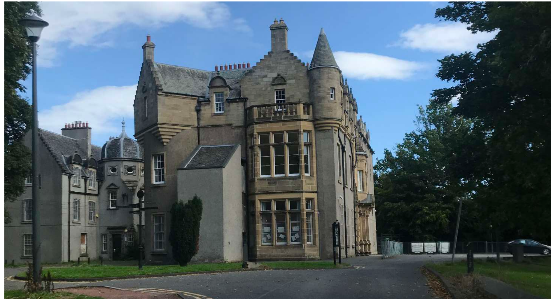
View from the west towards Inch House from the historic access drive
