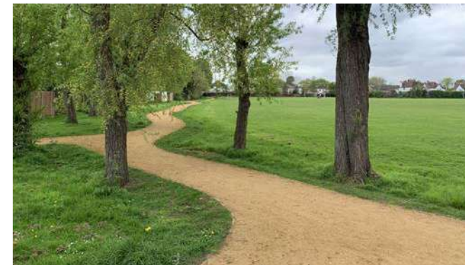
Breedon gravel / permeable surfacing to informal paths &amp; croft area
