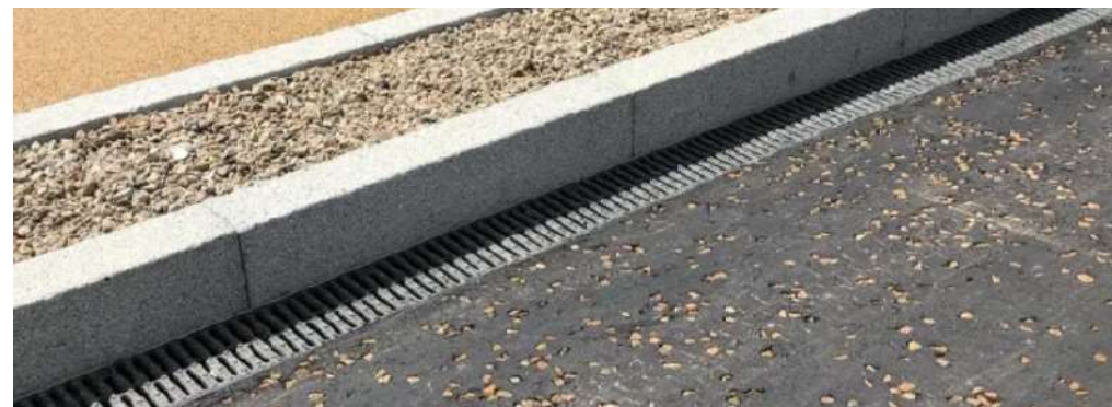
Hot Rolled Asphalt with buff chippings to parking and primary vehicular routes
